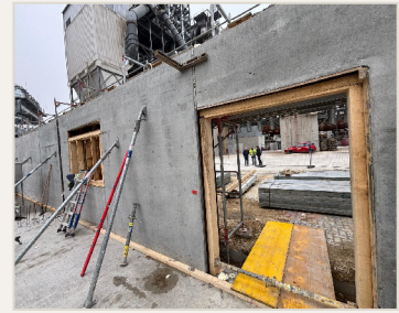
I-FOAM BUILDING UNDER CONSTRUCTION • MUNICH 2026
